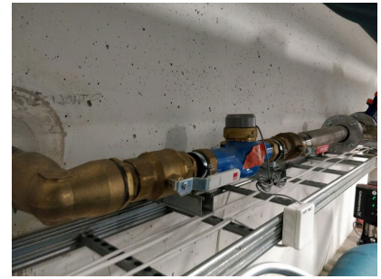
Water inlet shut-off
