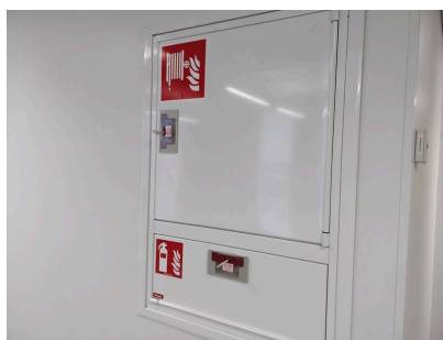
Fire extinguisher and fire hydrant
