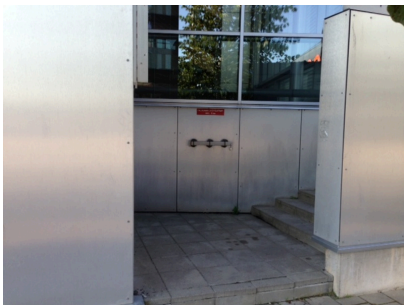
Additional water supply to the sprinkler system
