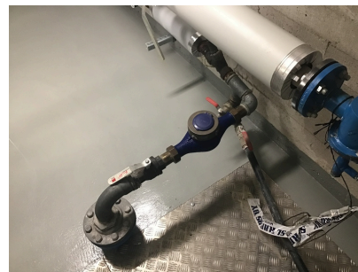
Water inlet shut-off in the heat room
