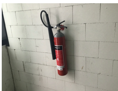
CO2 extinguisher for electrical and telecommunications rooms
