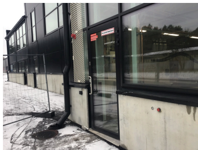
Access to the fire detector in the remote cold room and the pipe lock for the rescue service
