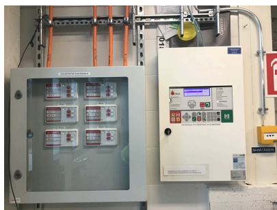
Fire alarm centre, remote smoke extraction and emergency stop button for ventilation in the remote cooling room
