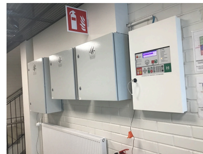
Smoke extraction units and fire alarm control panel in the corridor of stairwell 013b
